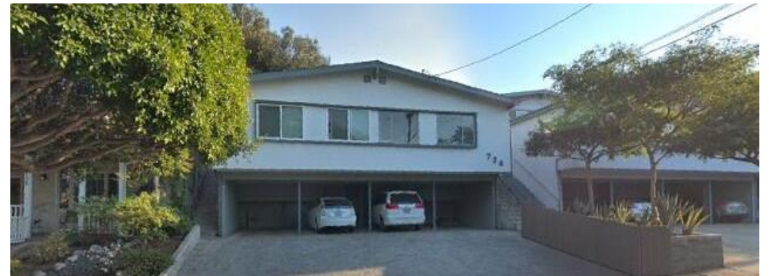
A typical soft-story building from google street view using Santa Monica DS
